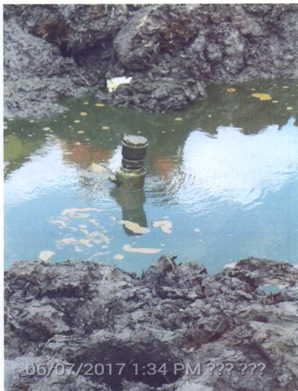
3" VALVE INSATALLED ON THE P/L
