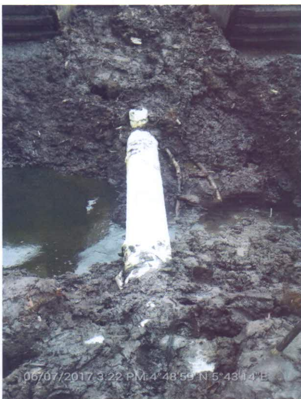
LEAK POINT REPAIRED
